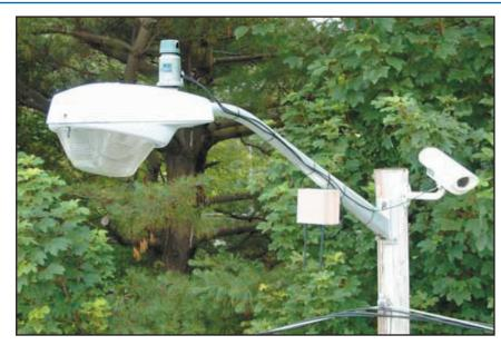
The AC to DC OWL provides DC power through a user specified cable and user specified connector for ancillary devices. The input power comes from a standard NEMA Street Light receptacle. Any line voltage up to 480 VAC is converted to user specified DC voltage.
